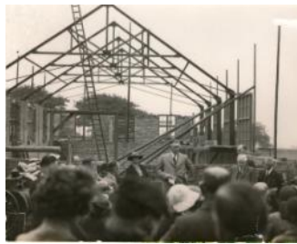
Building the Village Hall
